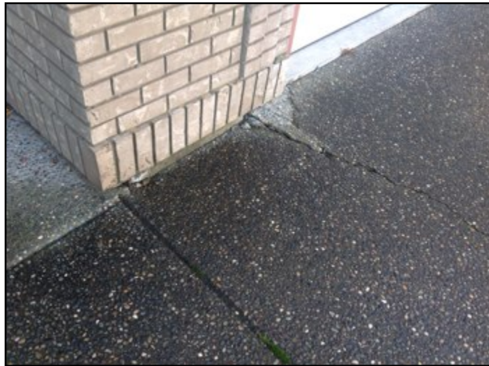
31. Cracked or damaged surfaces
