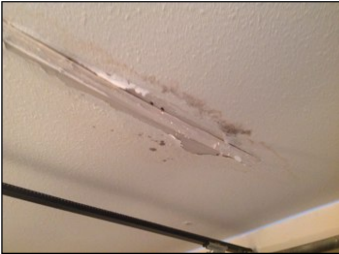
49. Water damage
