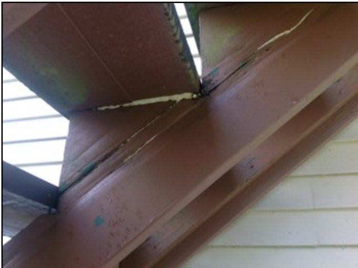
22. Rot or insect damage
