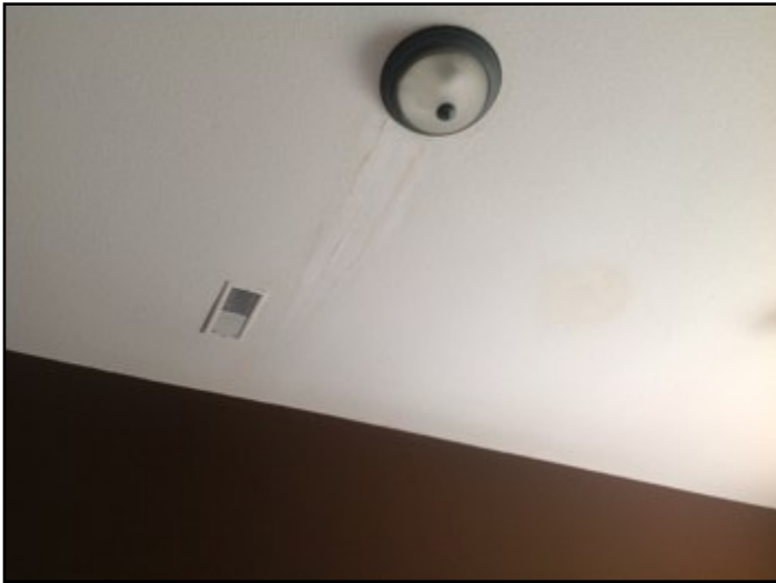
46. Water damage
