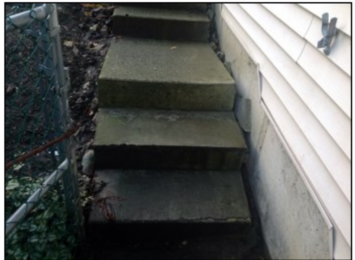
28. Steps or landings settling or heaving
