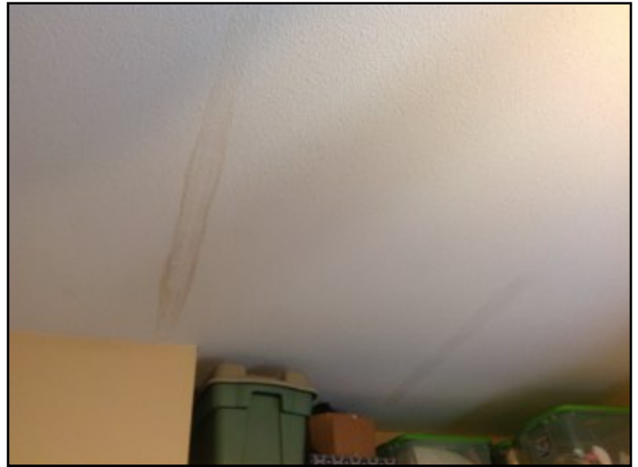
47. Water damage
