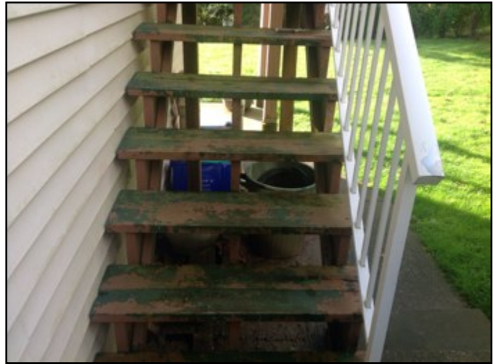
25. Rot or insect damage
