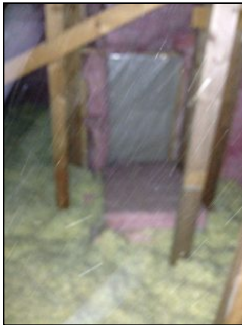
37. Inadequate in knee wall areas
