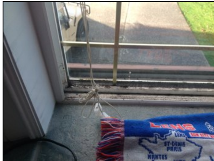
51. Clean window tracks of mold.
