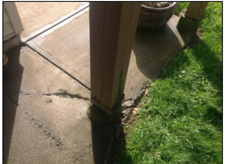
23. Rot or insect damage
